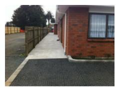
A decorative river pebble 5 - 10mm (discrete) was used for the filling and capping the **JakMat** *Geocell*.
